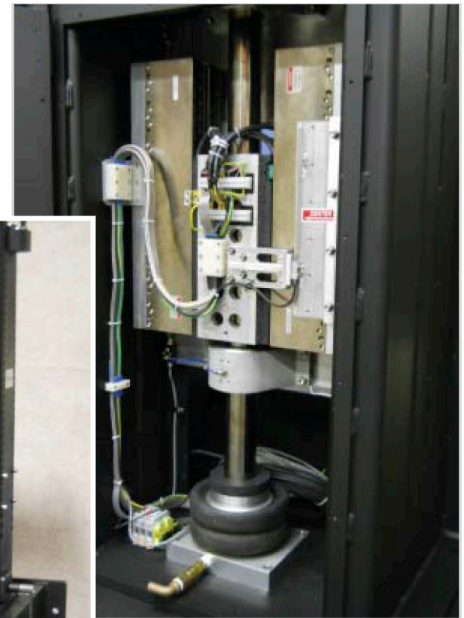
VIEW OF MOTORS & INSIDE FRONT
